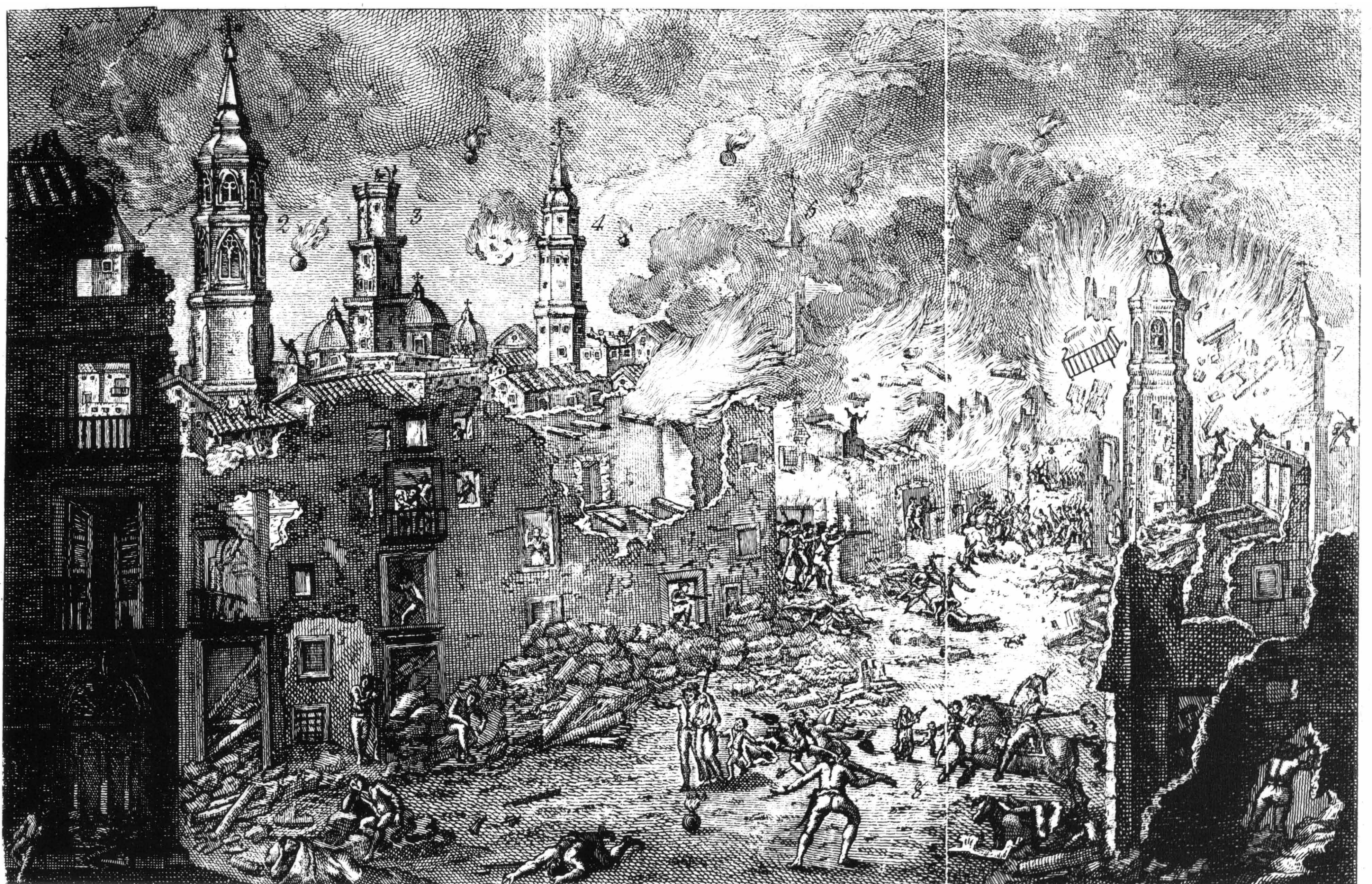
INTERIOR VIEW OF THE DESTRUCTION OF ZARAGOZA, IN THE SECOND SIEGE. 1 Parish church of San Pablo. 2 New Tower and Watchtower. 3 Our Lady of Pilar. 4 The Seo. 5 The Magdalena. 6 San Juan. 7 Santa Engracia. 8 Coso Street.
